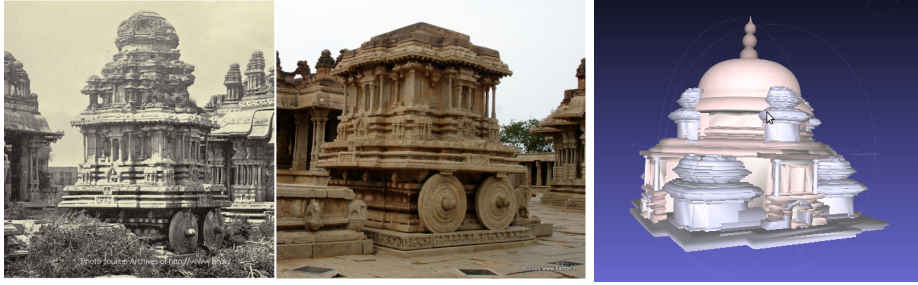
Fig. 8: The Heritage structure in 1856 (courtesy hampi.in ) and now. Note the dome-like superstructure that no longer exists. Fig. 9: The 3D model of the missing dome constructed by architects.
